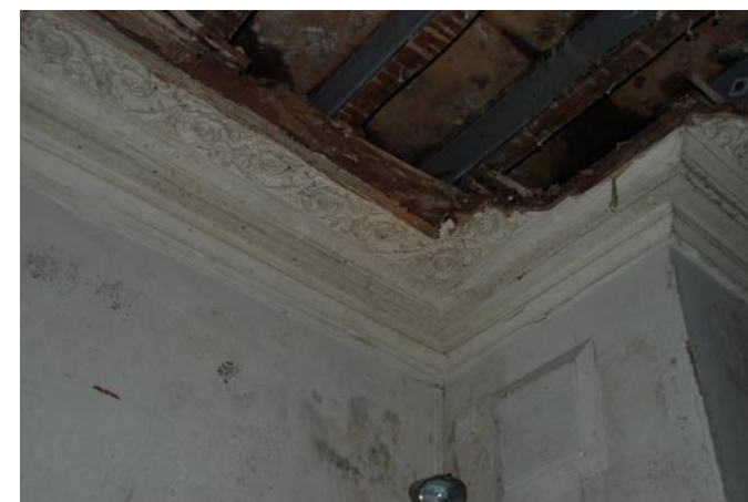
The only area of original plaster cornice remaining in the building is in the east wing ground floor area of the Main House.
