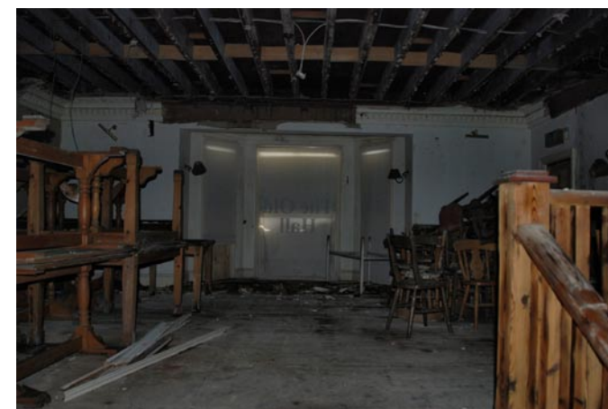
Floor levels were raised in the ground floor areas during the late 1960s alterations, which has resulted in a poor relationship with the window cill levels. It is proposed that these raised areas are removed and the original floor level reinstated. The ceiling and coving in this area is non-original.
