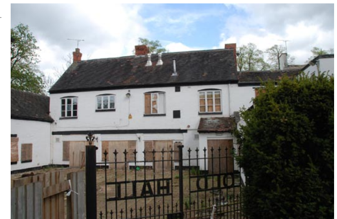
Two storey courtyard building (on east side of courtyard) appears to have been constructed between 188 and 1913. The ground floor was originally open sided with piers and was infilled in the mid 1990s
