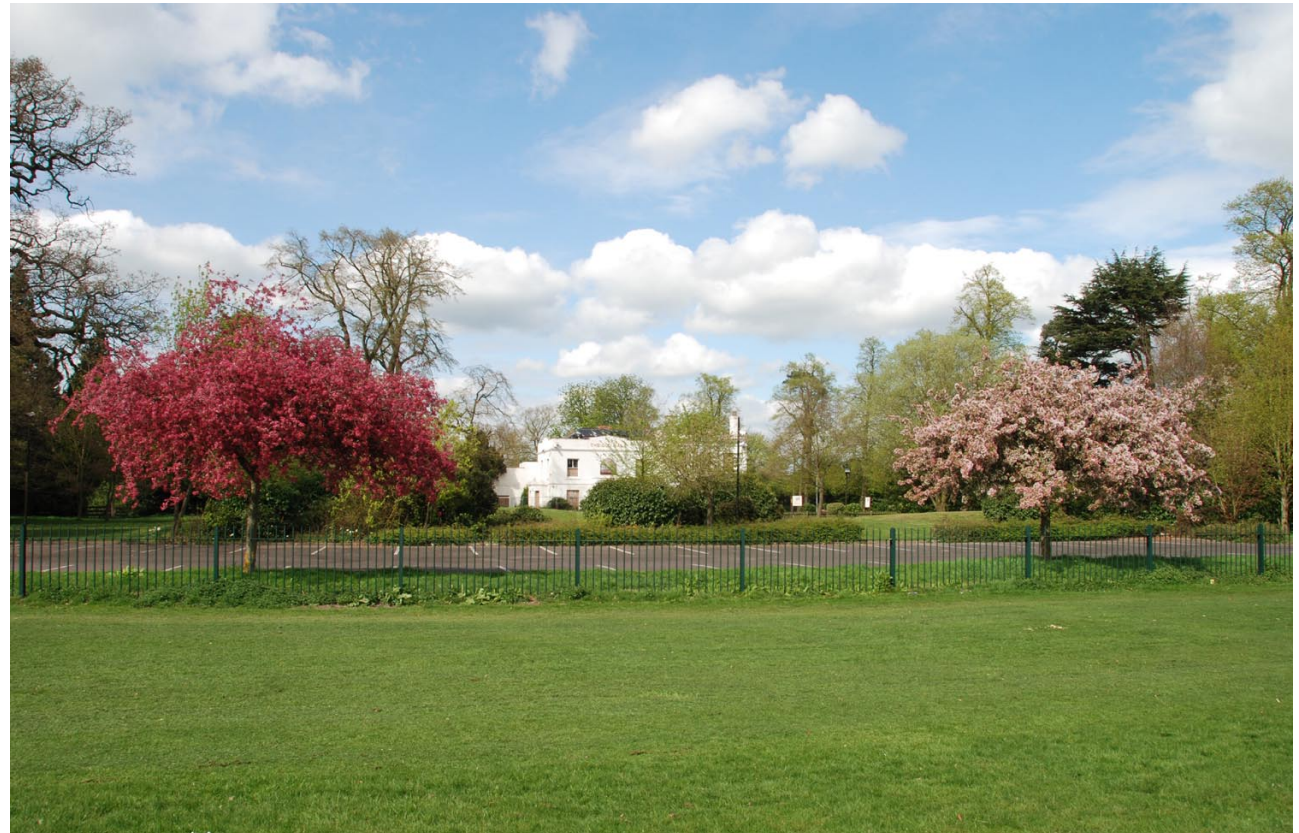
View looking north from Coundon Hall Park showing principal facade of Old Hall
